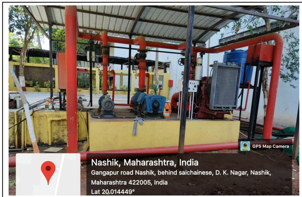
Central Water Tank
